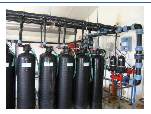
The catex unit with automatically operation is linked up to river water treatment
