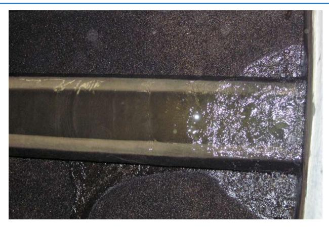
Clarified water from clarifier is run through the sand-filter, which catches remaining mechanical pollution
