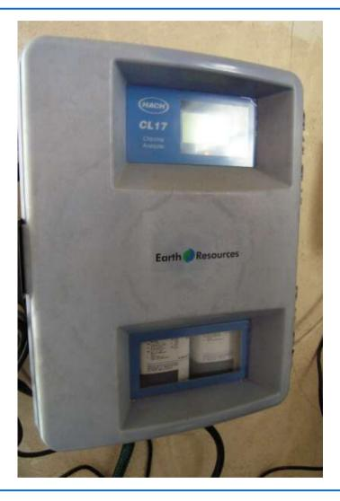
Control unit of the automatical dosage of sodium hypochloride, which ensures the microbiological quality of water
