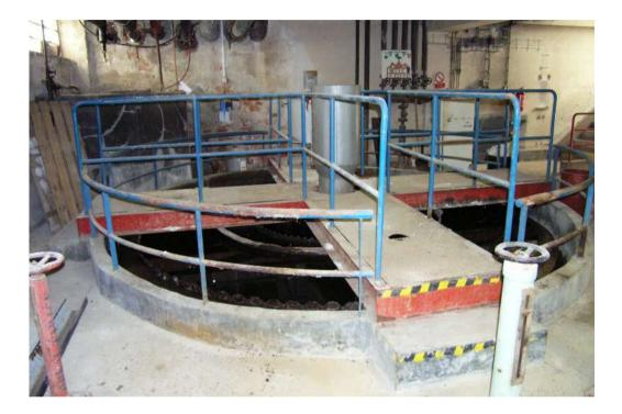
The river water is pumped into clarifier (see picture). By adding of aluminium sulphate and mixing are the Fe3+ and Mg2+ salts flocculated. The bulk of pollutions are rising to the water surface and mechanically removed.
