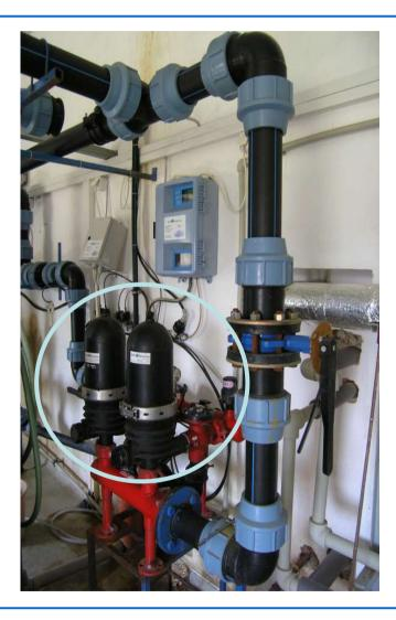
Disc water filters are equivalent to sand filters
