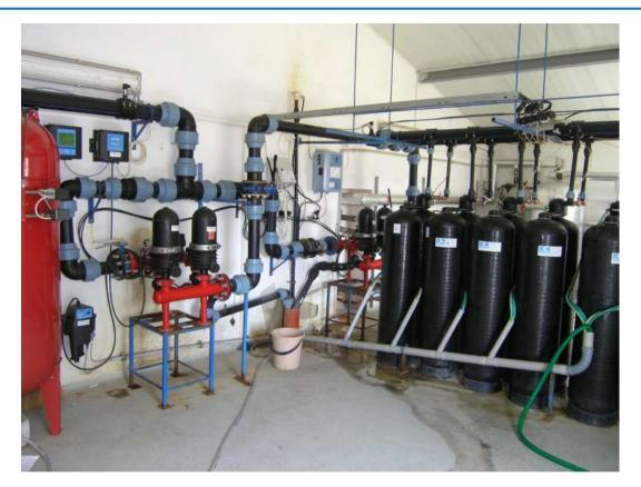
Overview of the water treatment unit – disk water filters, catex units and control unit for monitoring of water pollution
