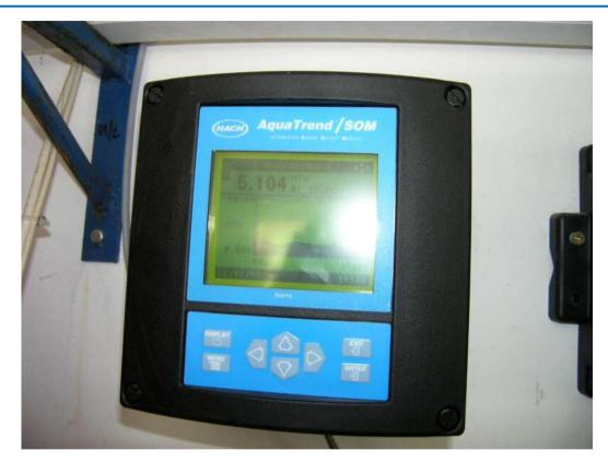
Water pollution is monitored by control unit – photometric monitoring of turbidity. When the limits are exceed, the unit switches the laundry to drinking water distribution.
